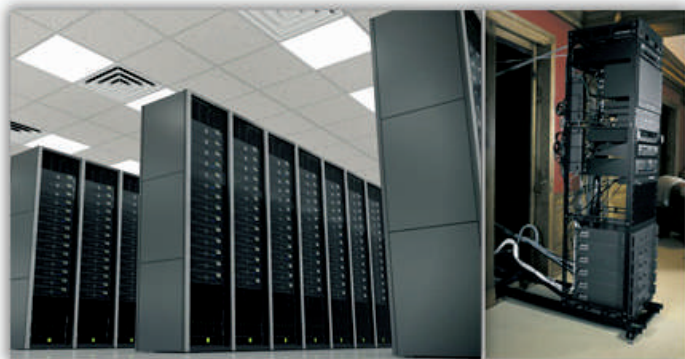
Servers - Rack & Sliding Server
